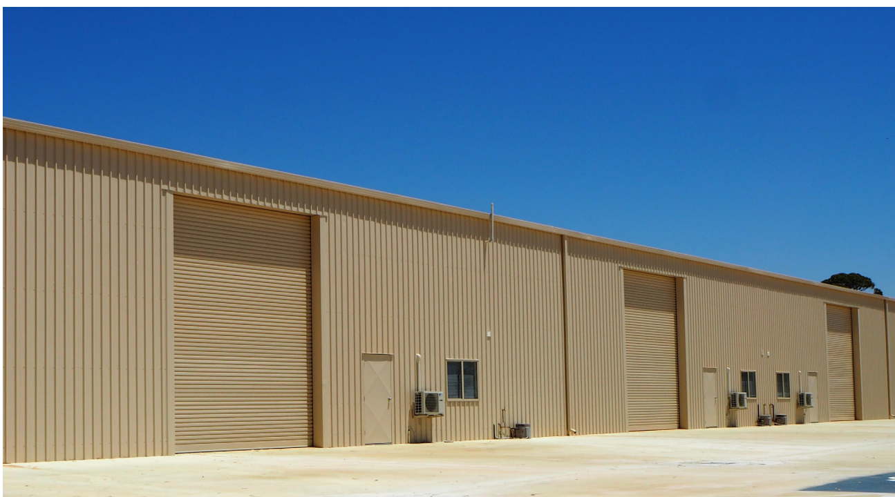
Industrial Factory Units built with Royalties for Regions Funding
