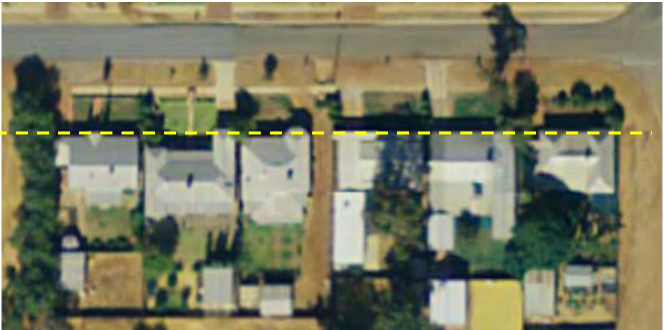
Existing Building Line (Street Setbacks) @ 36 – 46 McNeill Street, Dalwallinu (Landgate)
