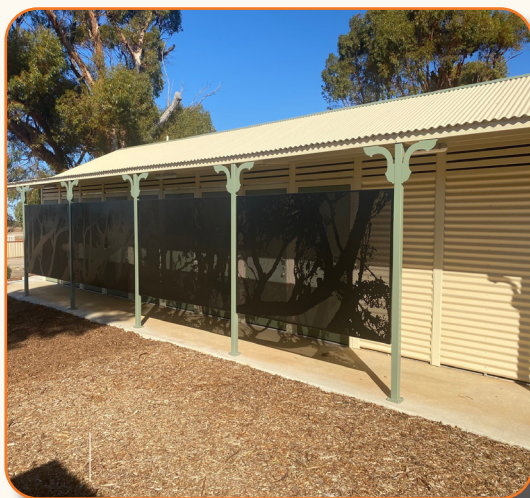
New Ablutions, Dalwallinu Caravan Park
