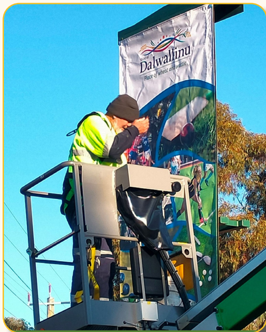
Installation of sports precinct banner using new cherry picker
