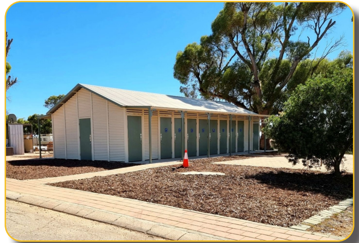
Dalwallinu Caravan Park - new ablutions block
