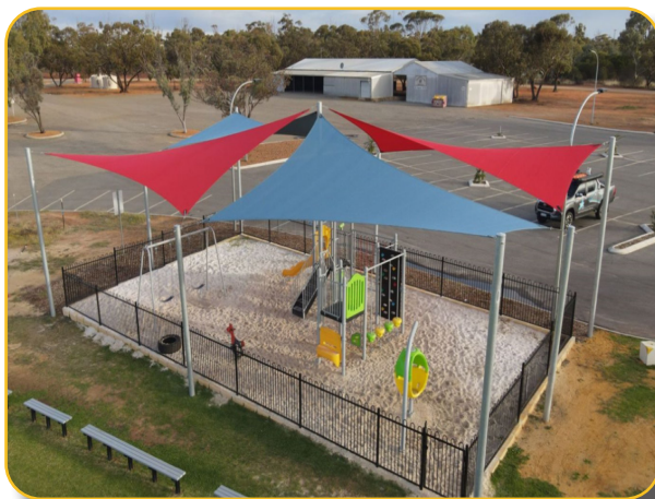
Dalwallinu Recreation Playground - new shade sails
