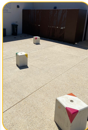
Block Bollards - Dalwallinu Recreation Centre
