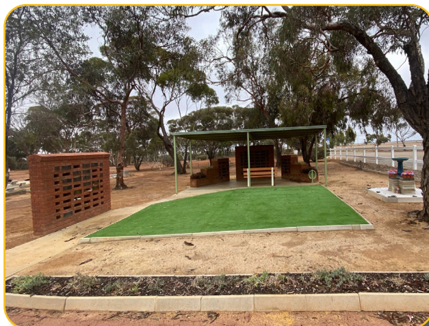
Dalwallinu Niche Wall - new works
