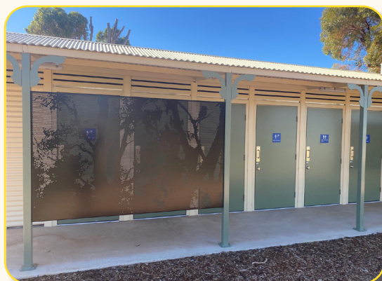
New Ablutions Block - Dalwallinu Caravan Park
