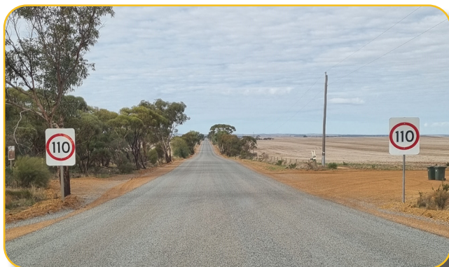
Dalwallinu-Kalannie Road - new seal
