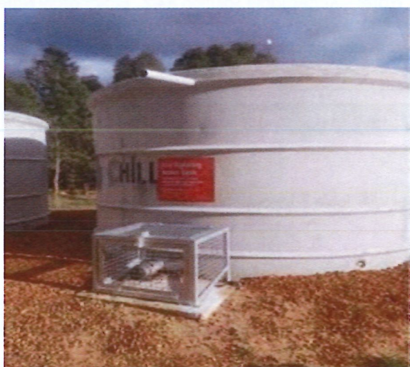
Strategic 47,000 Litre Concrete Tank & Protected Fittings
