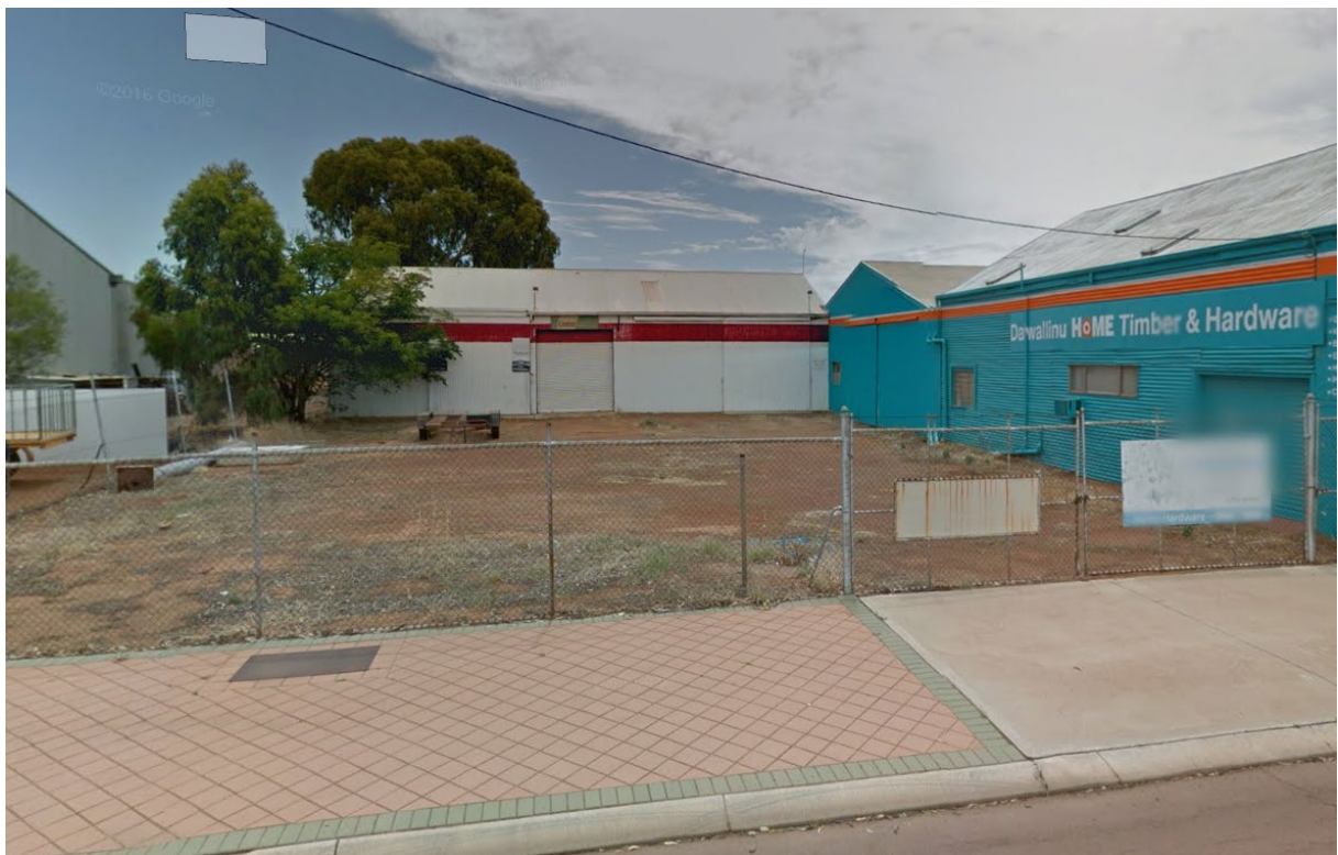
Street View of Subject Premises (googlemap)
