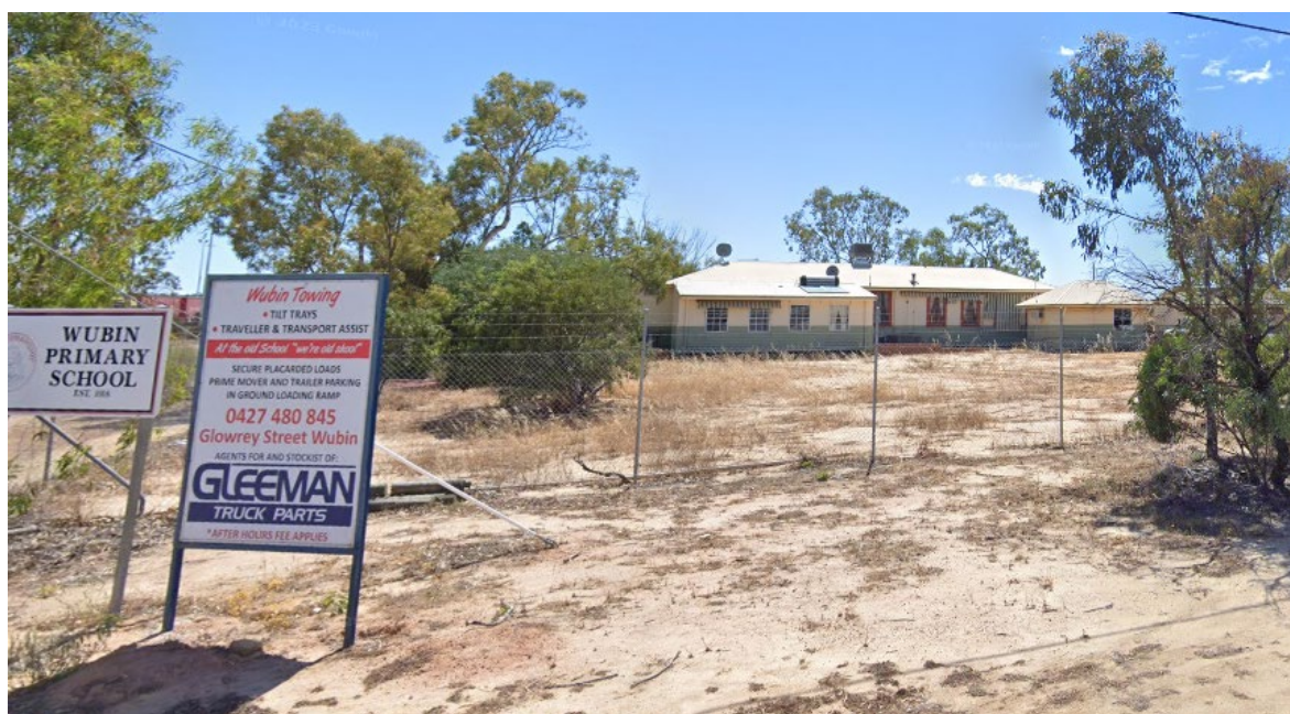
The subject property from a North-west aspect
