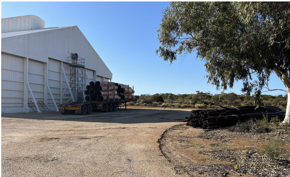
The subject property from a North-west aspect
