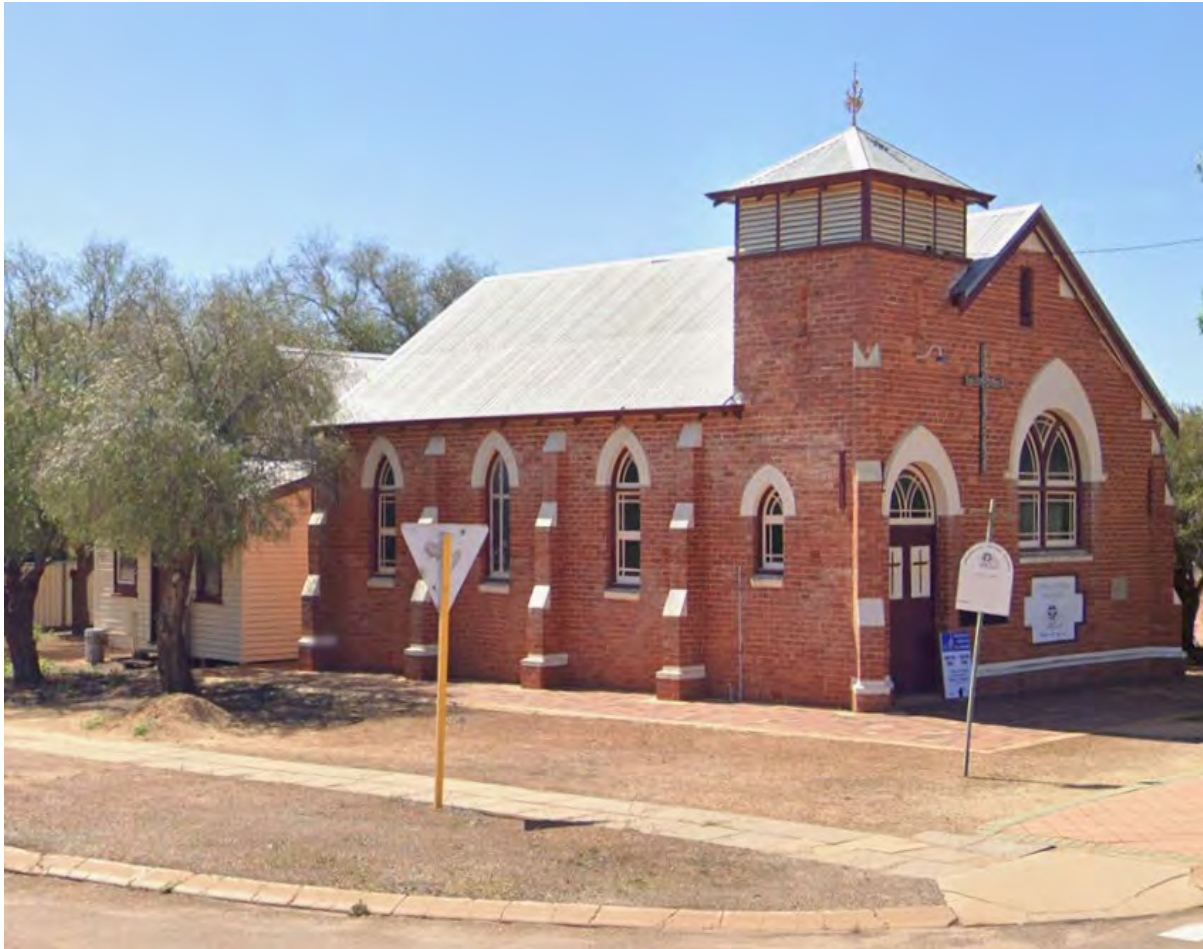
Street view of Lots 139 & 140 McNeill Street, Dalwallinu (Google Maps)
