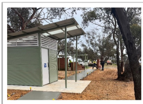
New Ablution Block Dalwallinu Cemetery
