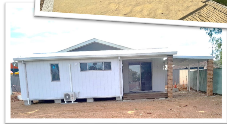
New Emergency Accommodation Housing
