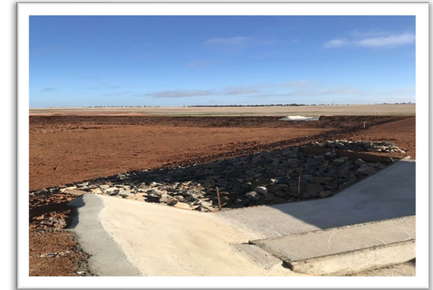
Annetts Road Stormwater Catchment
