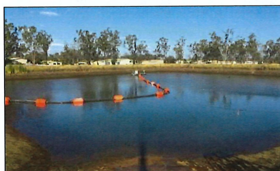
Figure 3. Six-inch on water pipework and floats
