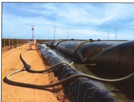
Figure 1. Dredged sludge being dewatered via Envitube® geotextile dewatering containers.
