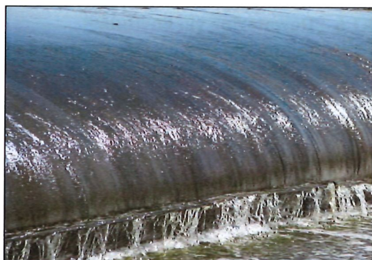
Figure 2. Clear filtrate flowing through the geotextile fabric
