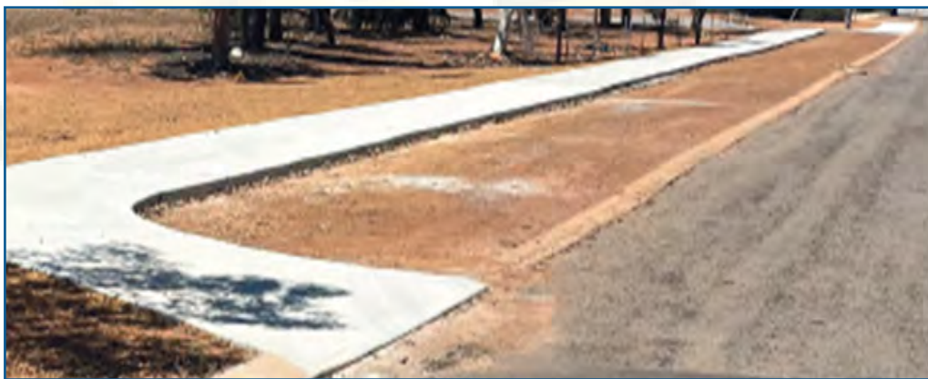
Owens Avenue footpath extension
