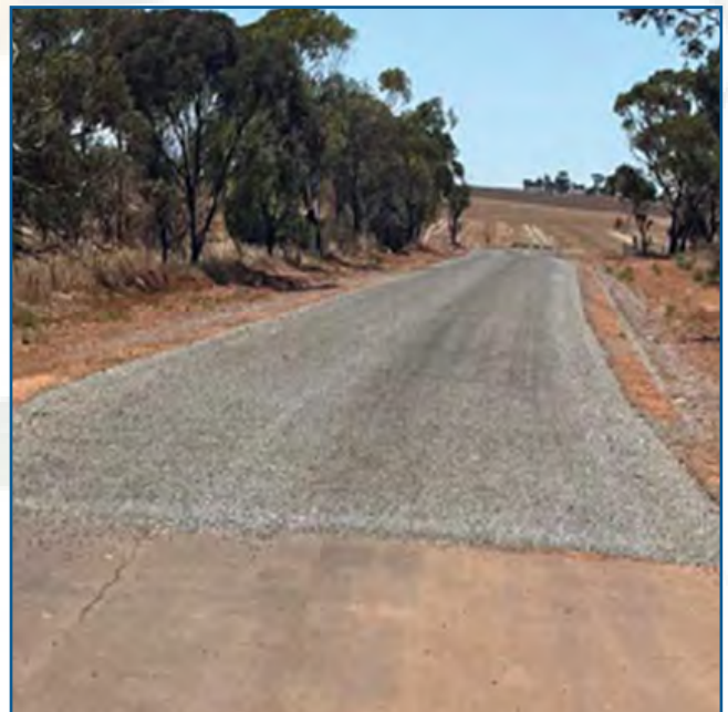
Continuation of seal on Annetts Road
