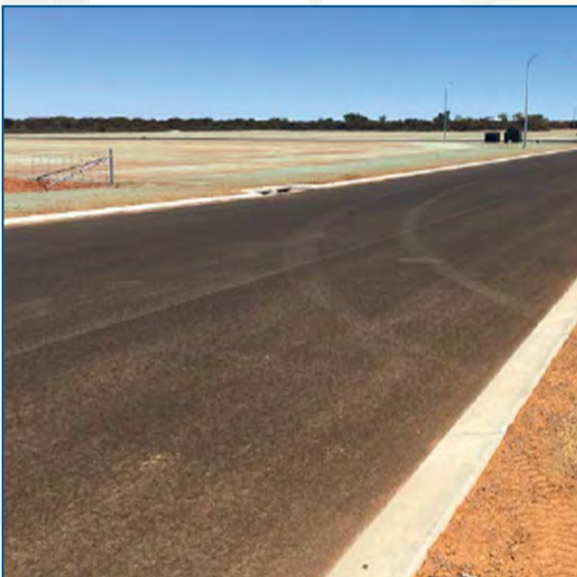
New industrial division extension
