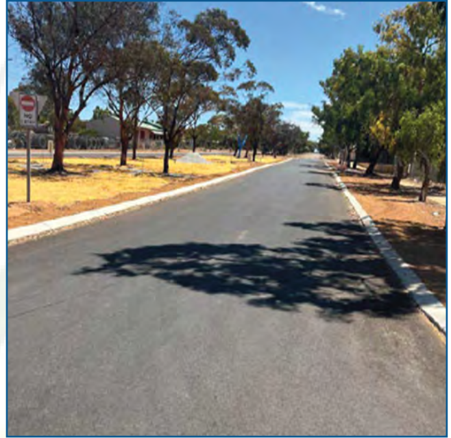
Leahy Street new kerbs and seal looking west
