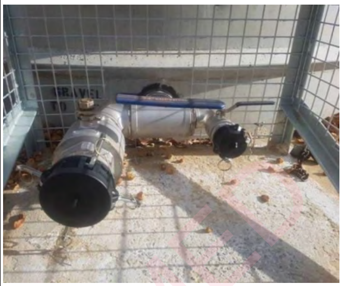
Strategic 47,000 Litre Concrete Tank & Protected Fittings
