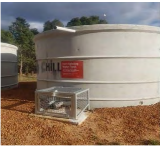
Strategic 47,000 Litre Concrete Tank & Protected Fittings
