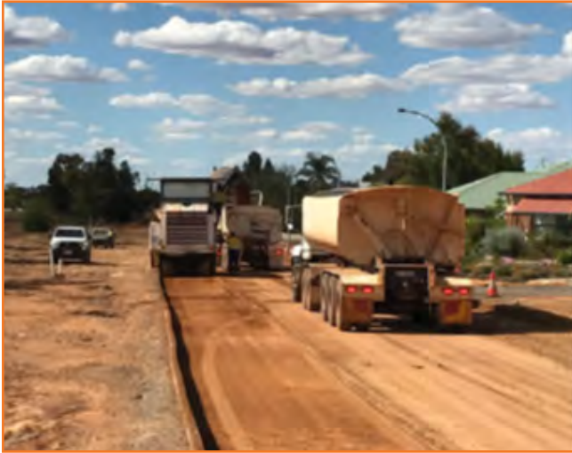
Annetts Road Reconstruction
