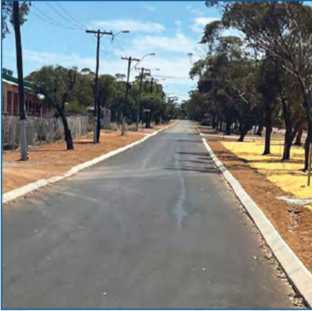
Leahy Street new kerbs and seal looking east
