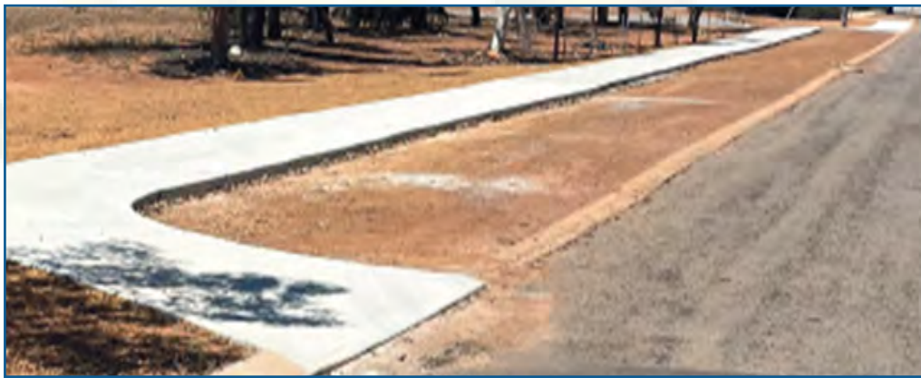
Owens Avenue footpath extension
