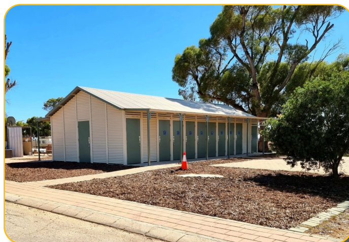
Dalwallinu Caravan Park - new ablutions block
