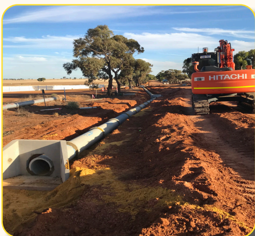
Roberts Road - under construction
