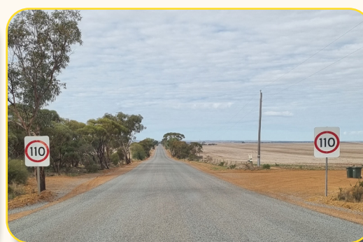
Dalwallinu-Kalannie Road - completed
