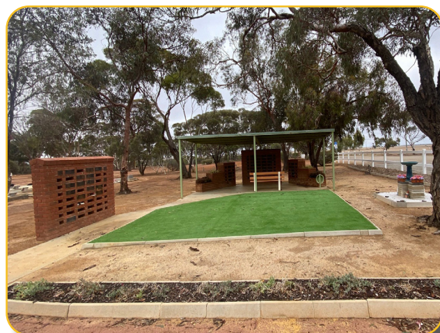
Dalwallinu Niche Wall - new works
