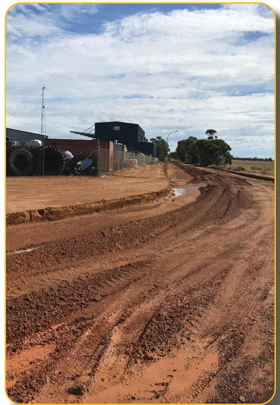
Roberts Road, Dalwallinu - new road construction
