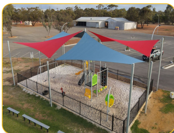
Dalwallinu Recreation Playground - new shade sails
