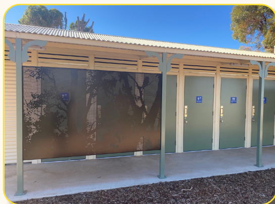
New Ablutions Block - Dalwallinu Caravan Park
