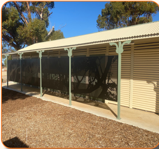
New Ablutions, Dalwallinu Caravan Park
