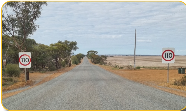
Dalwallinu-Kalannie Road - new seal
