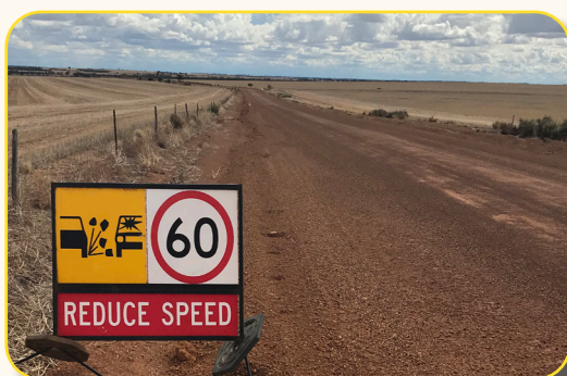
Dalwallinu-Kalannie Road - under construction
