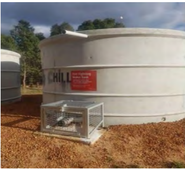
Strategic 47,000 Litre Concrete Tank & Protected Fittings
