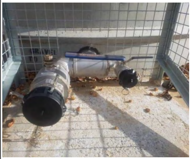
Strategic 47,000 Litre Concrete Tank & Protected Fittings
