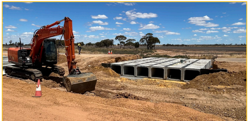
Reconstruction and culvert works have begun on Dowerin-Kalannie Road. The Shire installed the culverts and Fulcher Contractors are the contractors completing the road works.
