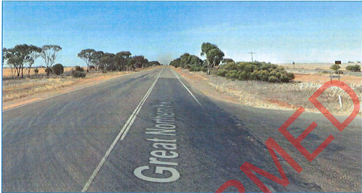
Figure 7: CBH Access Road/GNH Intersection - Looking South
