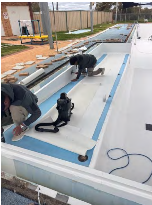
Geotextile being installed along with new PVC Liner
