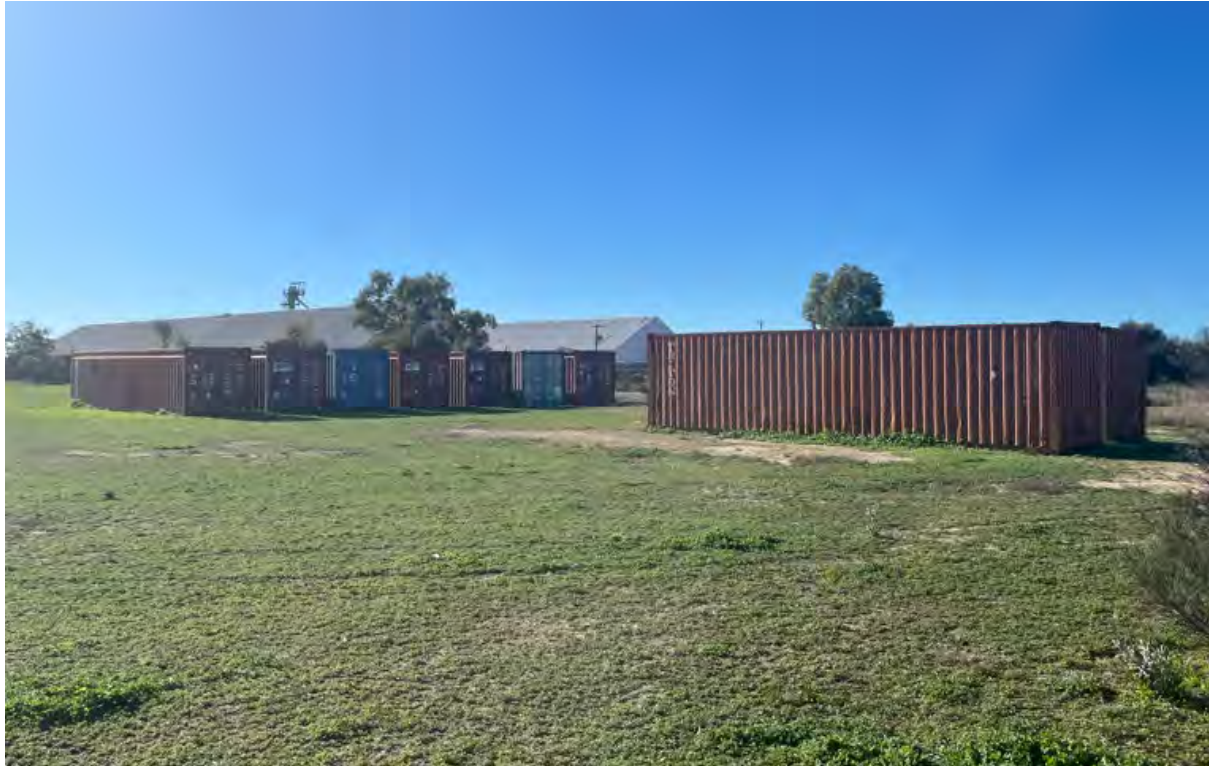
Shipping containers on Lot 506 Harris North Road, Wubin
