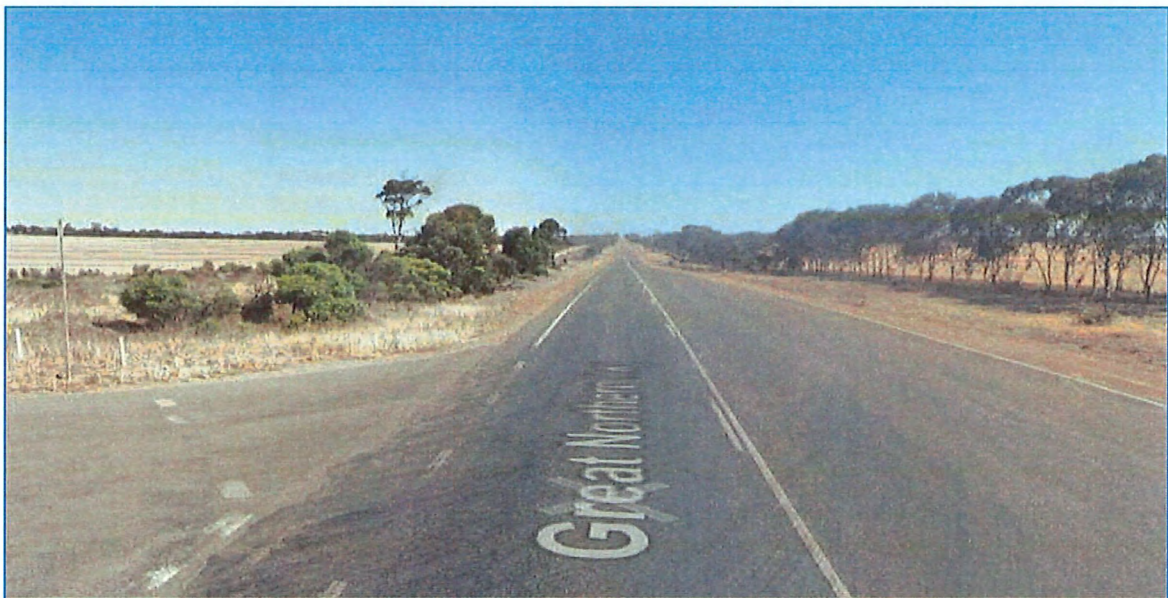
Figure 8: CBH Access Road/GNH Intersection – Looking North
